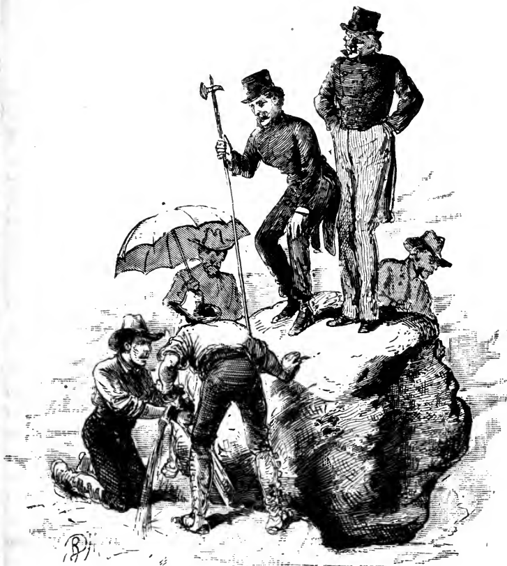
SPRUNG A LEAK.
