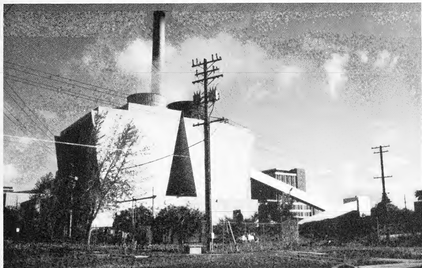
Fig. 2a. A University of Wisconsin heating plant.
