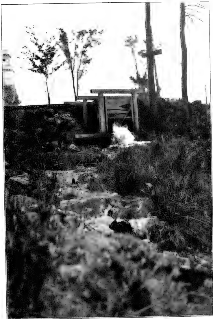
DAM-POND No. 2 AND BROOK BETWEEN PONDS No. 2 AND 3.
