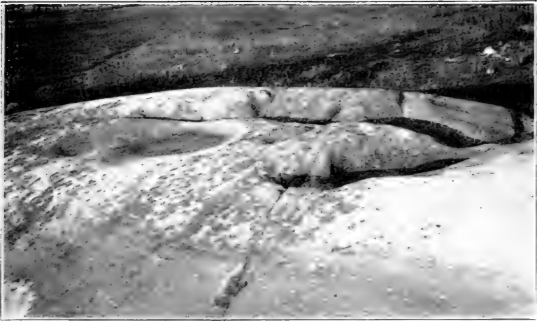
Fig. 3. Potholes due to removal of granite sheeting slabs.
