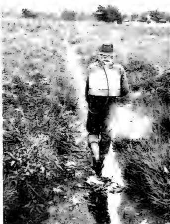
Oiling a cleared ditch to kill mosquito wigglers.
