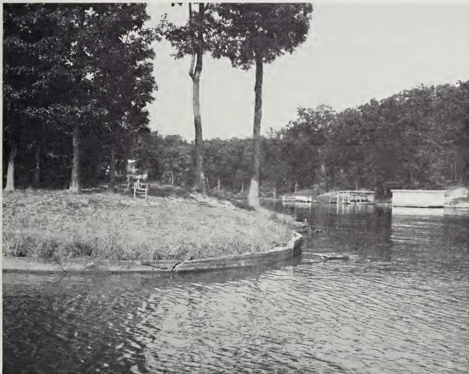
FIGURE 6a. Wall failure where reinforcing rods were omitted.
