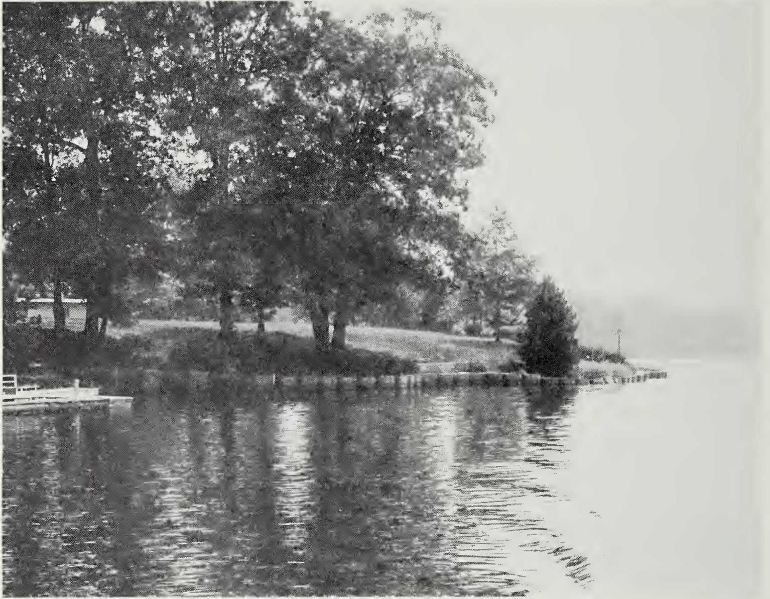
FIGURE 6b. Corrugated area-way projections provide strength to erosion barrier.
