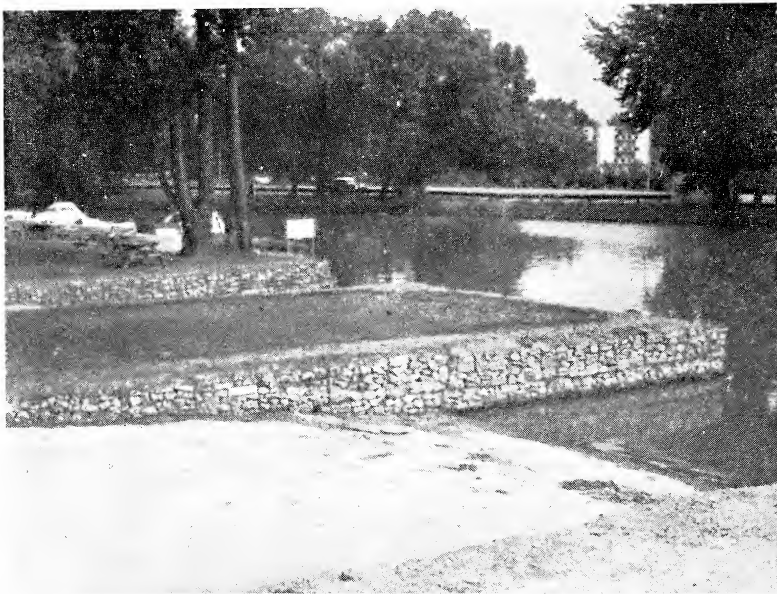
FIGURE 8. This gabion wall protects lake-front property.
