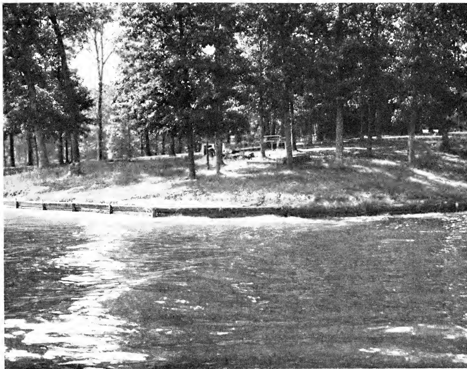
FIGURE 2. Low wood barrier wall.
