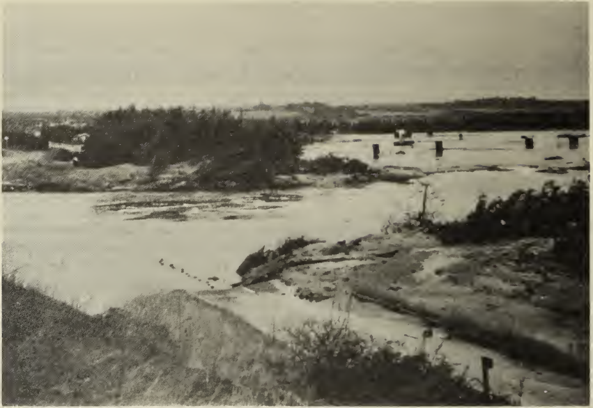
Fig. 1. The second breach in the Sea Wall, photographed on 15th January. This was the breach nearest the "Orchidetum", and also shows where a whole section of the 20 year old Pines was swept away.
