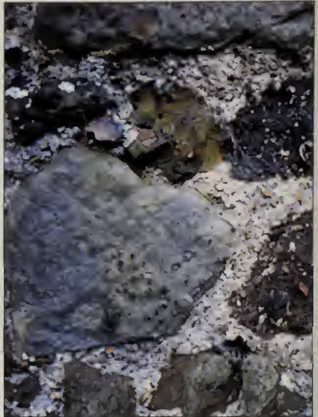
A piece of the wall of South Wootton church, showing a variety of local building materials, including dark gravelly ferricrete, local white sandstone and flint.
