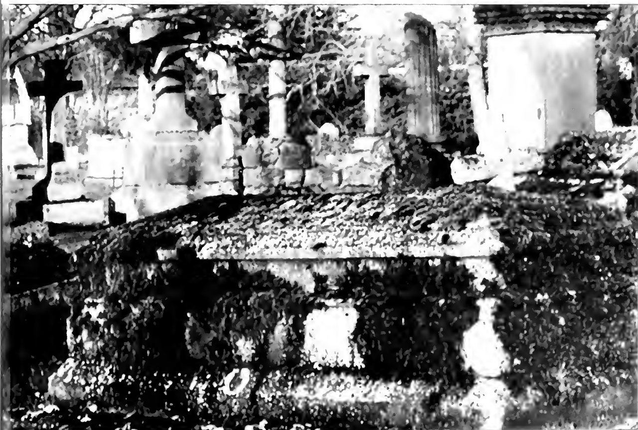
This variant of the Box or Chest tomb has gently sloping upper surfaces. Made of oolite, it has acquired a rich covering of moss.
