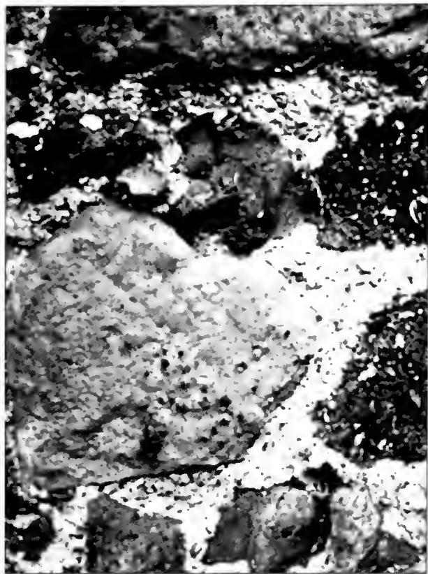
A piece of the wall of South Wootton church, showing a variety of local building materials, including dark gravelly ferricrete, local white sandstone and flint.
