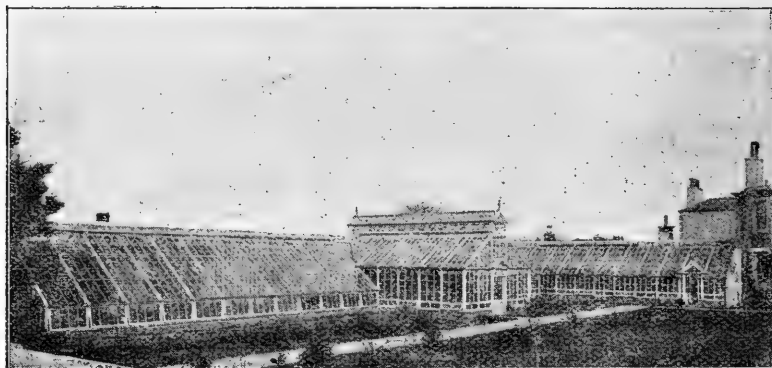
Range of Hothouses erected at St'Marnocks, Malahide.
