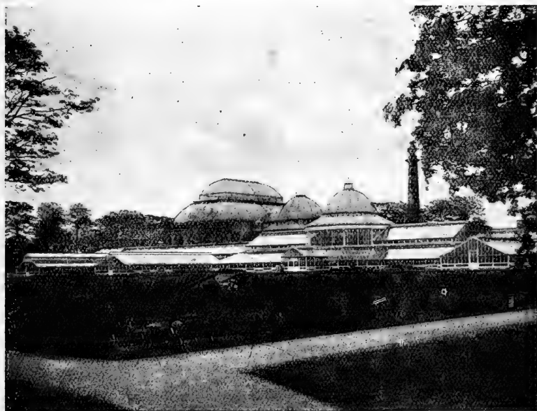
Plant Houses erected at Royal Botanic Garden, Edinburgh.
