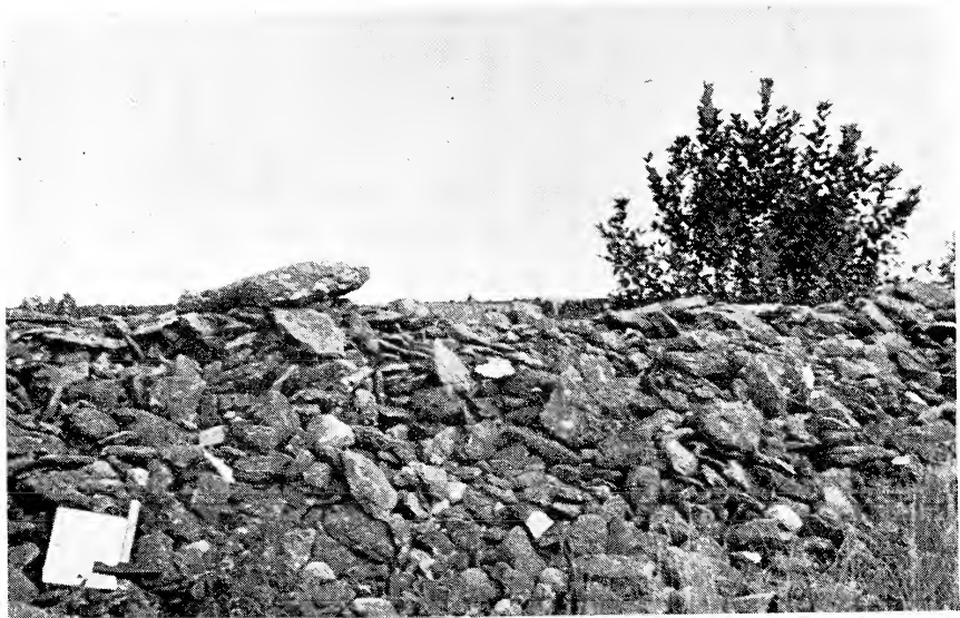
PLATE VI.—Rock fence along Highway 57 in Section 20, T31N, R28E.
