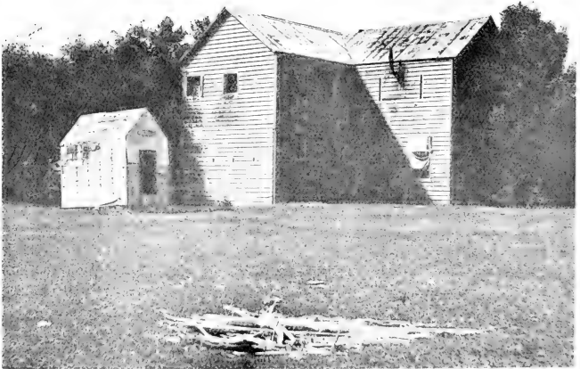
FIG. 2.—Old blockhouse near Wallaceville, built in 1860-61. Photo by J. McDonald, 1916, taken from a point near the bastion, and within the area originally stockaded. The timber lying in the foreground covers the mouth of the well.
