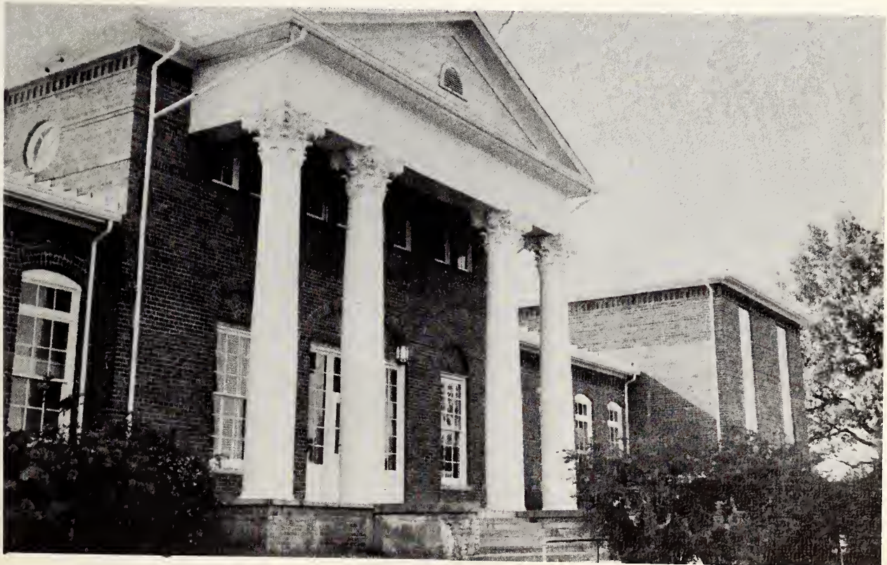
NORWOOD SCHOOL AUDITORIUM
