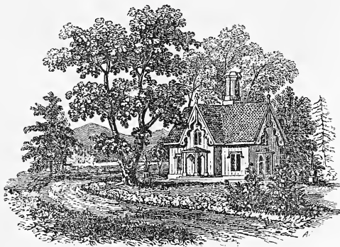
[Fig. 60. The Gardener's House, Blithewood.]
