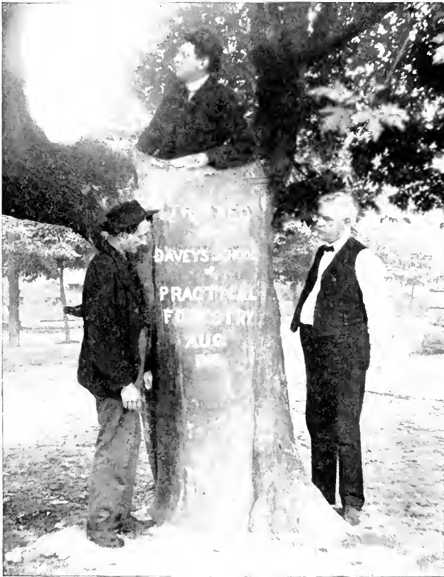
Photo 51 The Maple Filled and Finished.
