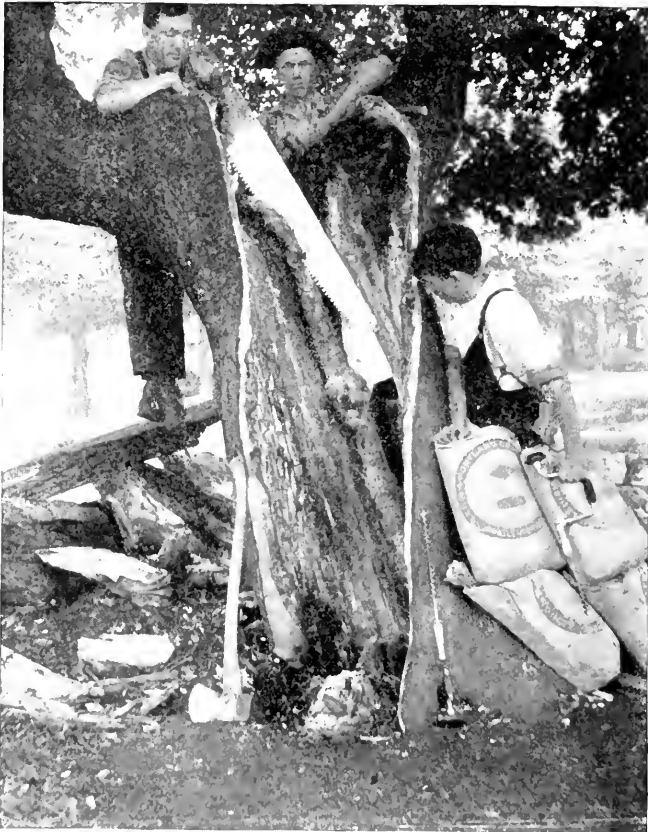
Photo 50 The Maple with Decayed Center partly Removed.
