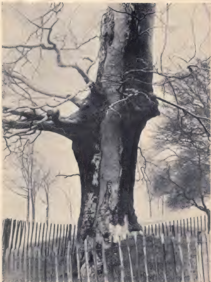
REPAIRING A BEECH TREE.
