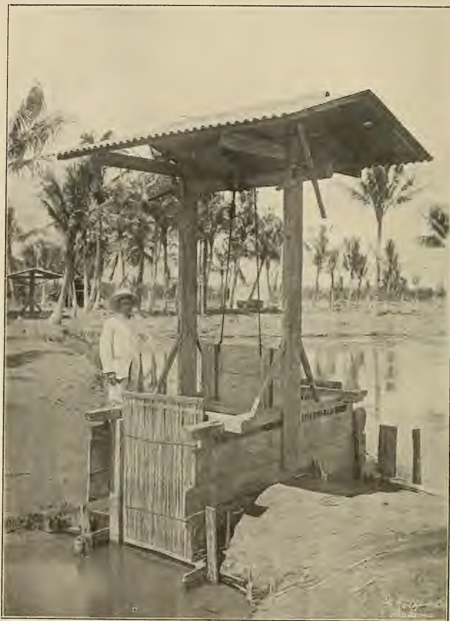
Photo no. 1. (Taken in 1915). Little sluice gate connecting two Batavia sea-fish-ponds, Pondsystem of Ang Sun Hian, Groningsche weg near Kampong Fluit (cf. Map I).
