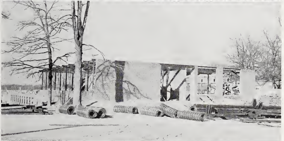
NEW HIGH SCHOOL BUILDING UNDER CONSTRUCTION
