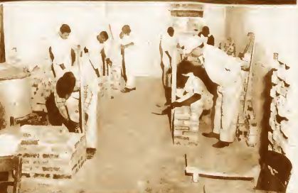
Mr. Hams' second-year masonry class is building yellow and solid piers of various sizes
