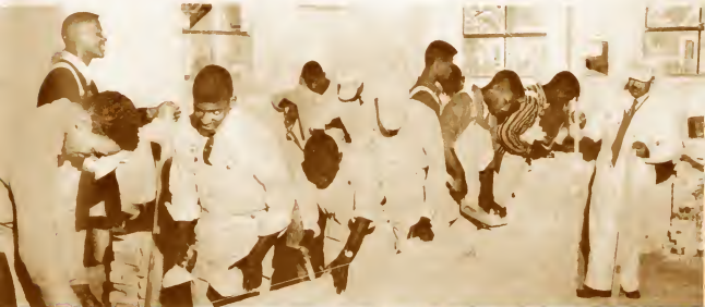
Mr. Harris' first-year masonry class is building eight-inch return corners and an eight-inch wall to the line.
