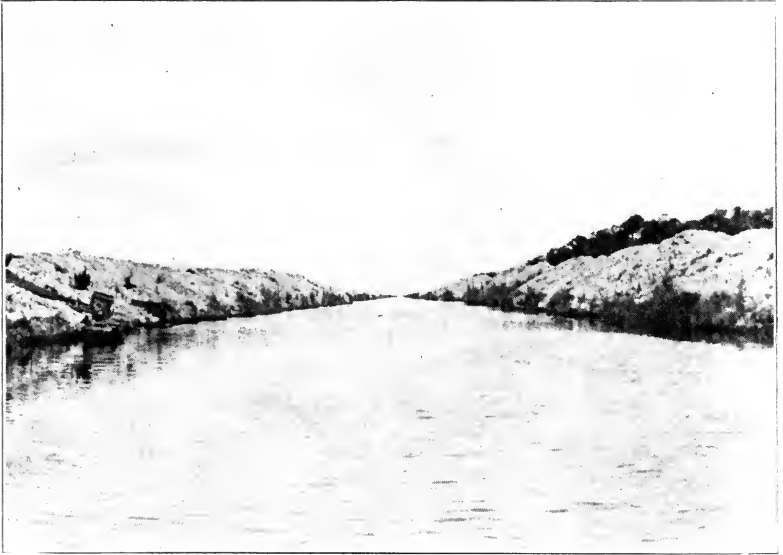
STATE CANAL IN THE EVERGLADES, FOR DRAINAGE, IRRIGATION AND TRANSPORTATION.
