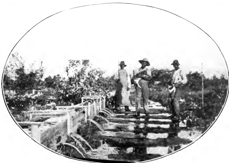
TROUGH FOR SURFACE IRRIGATION.
