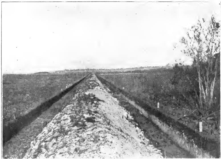
DYKE AND LATERAL DITCHES ON MR. WALDIN'S EVERGLADE FARM.
