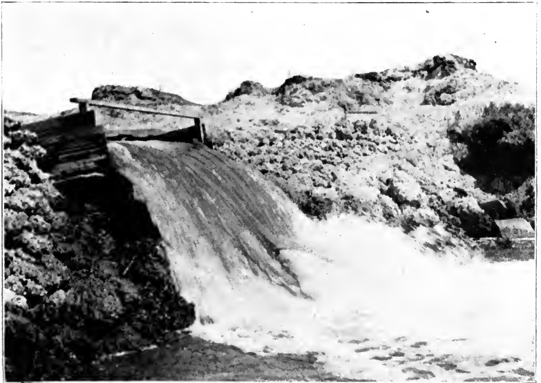
TEMPORARY DAM IN STATE CANAL, TO BE REPLACED LATER BY PERMANENT LOCKS.
