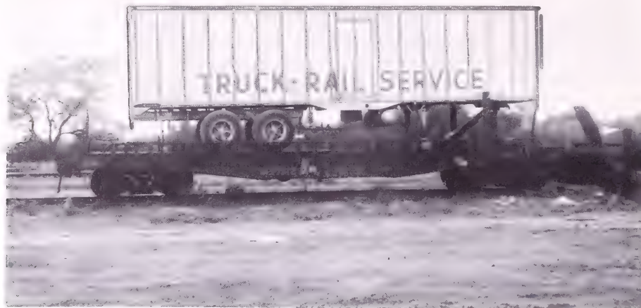
Figure 1. --Truck-rail series R or RF trailer loaded on flatcar. Single gangway at diagonal ends of car in raised position for transit.
