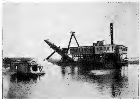
One of 20 dredges that cut over 600 miles of water-ways in Florida suitable for transportation, irrigation and drainage.
