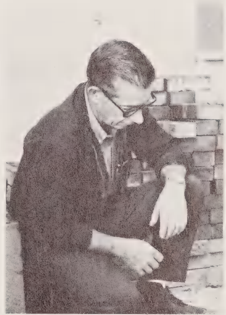
William Massey Bricklaying
