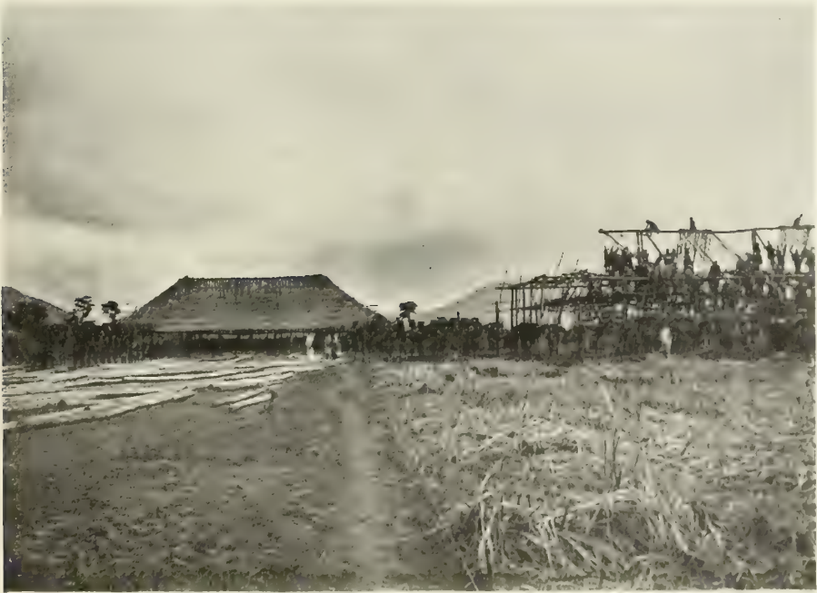
192. "GOVERNMENT HOUSE" AT HOMIA, UNYORO, IN PROCESS OF BUILDING.
