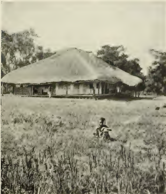
194. THE AUTHOR'S BUNGALOW ("COMMISSIONER'S HOUSE") AT ENTIBBI, BUILT BY MR. SPIRE
