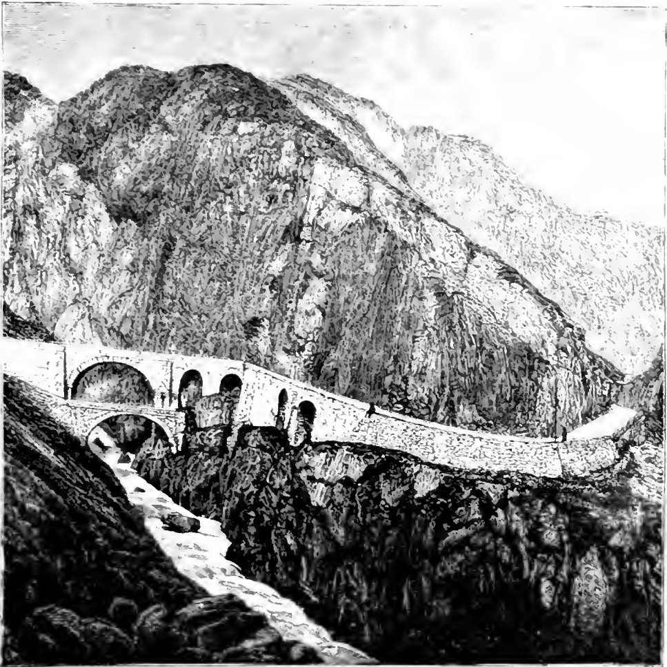
Fig. 329.—THE DEVIL'S BRIDGE AND THE ROAD OF THE ST. GOTTHARD.
