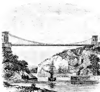
Fig. 66.—CLIFTON SUSPENSION BRIDGE.
