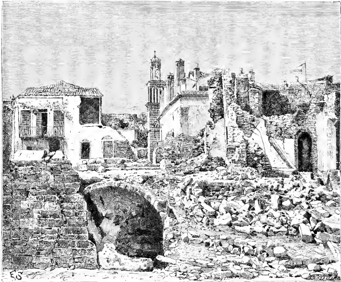
Fig. 136.—CHIO—VIEW TAKEN AFTER THE EARTHQUAKE OF 1881.
