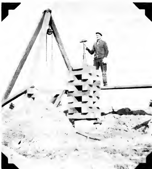
A. Screw jack working against anchored cable, forcing soil tank 6 feet into the ground to capture undisturbed soil.
