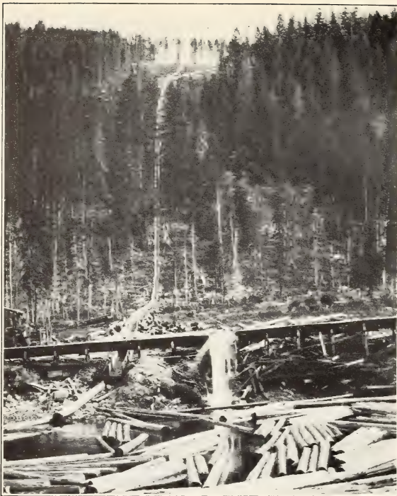
FIG. 1.—CHUTE DOWN WHICH LODGEPOLE-PINE STULLS AND OTHER MATERIAL ARE BROUGHT TO RESERVOIR IN FOREGROUND, DEERLODGE NATIONAL FOREST.
