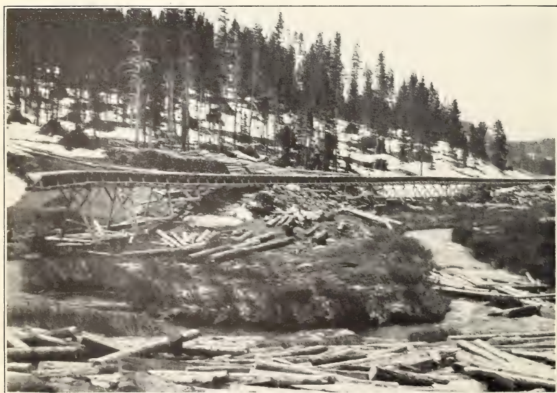
FIG. 2.—FLUME FOR TRANSPORTING LODGEPOLE-PINE TIES, PROPS, AND SLABBED LOGS, BIGHORN NATIONAL FOREST.
