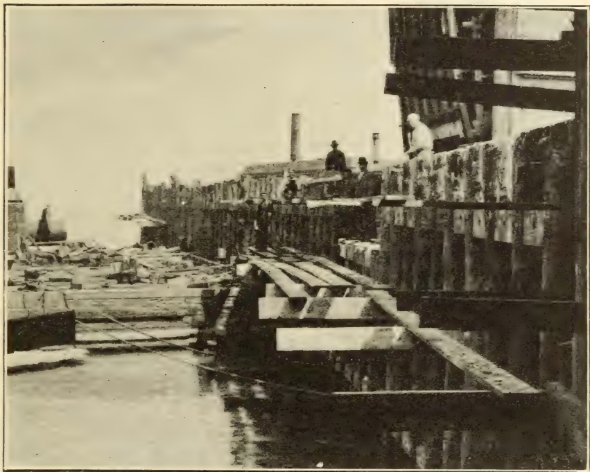
FIG. 6.—A ferry slip, San Francisco, Cal., constructed of blue-gum piles.
