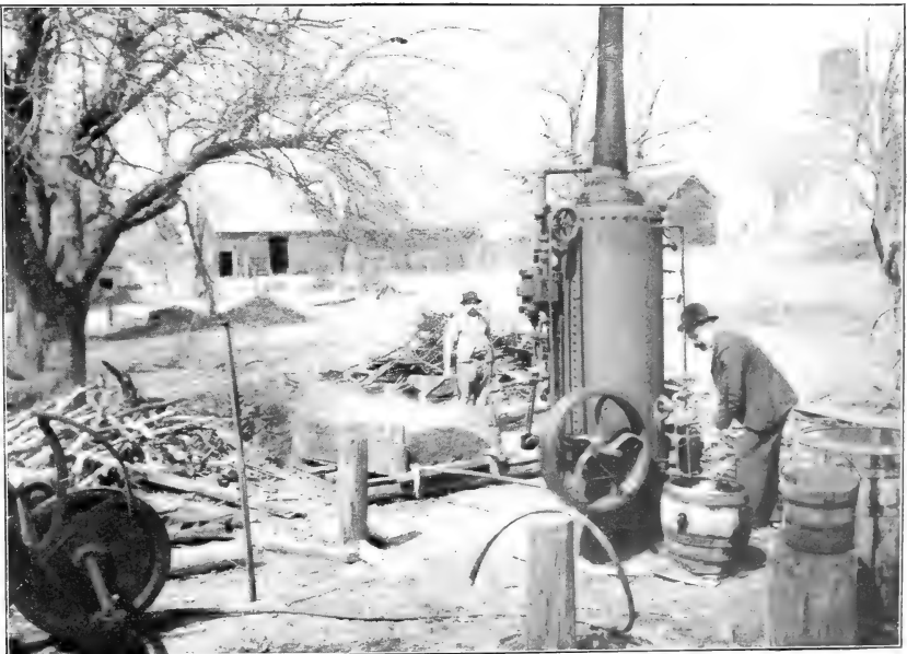
FIG. 2.—STERILIZING SOIL FOR TOBACCO SEED BEDS.
