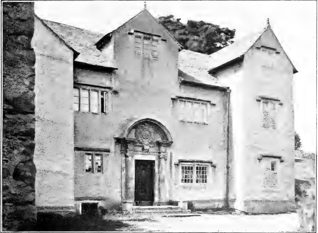
LOWER HOLKER : CARK HALL, FRONT VIEW
