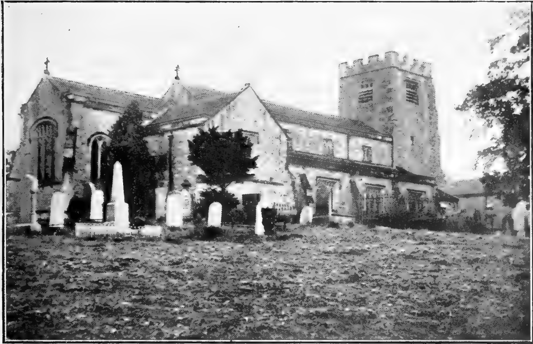
CATON CHURCH FROM THE NORTH-EAST
