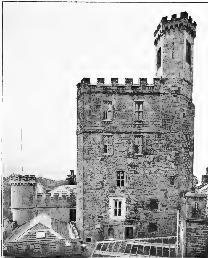
HORNBY CASTLE: NORTH SIDE OF TOWER FACING COURTYARD
