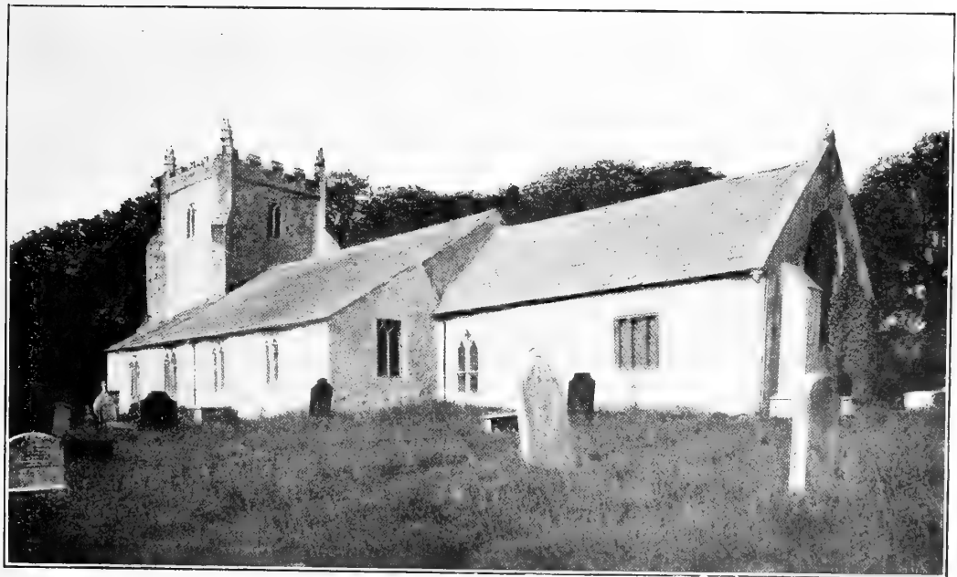
ALDINGHAM CHURCH FROM THE SOUTH-EAST
