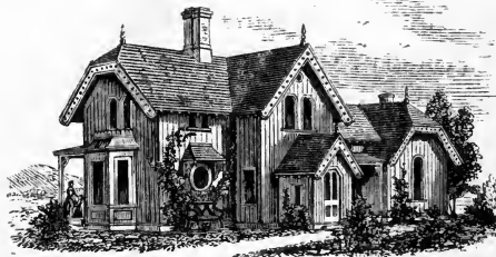
N.E. VIEW. SHOWING THE COTTAGE COMPLETED.
