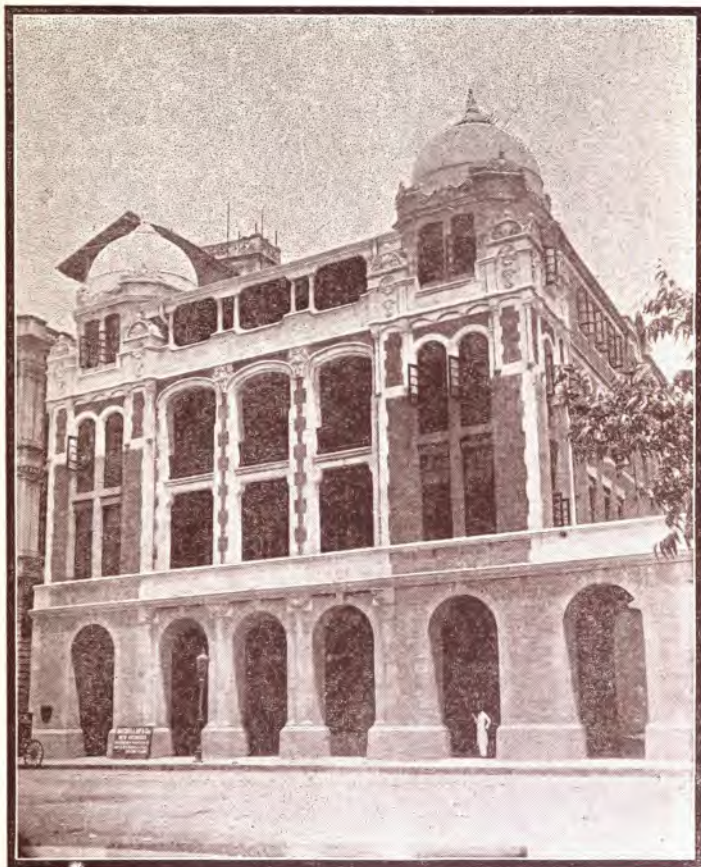
MACMILLAN'S BUILDING, HORNBY ROAD.
