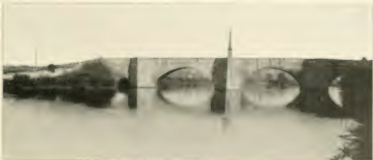
View from the bridge at Fozzoo.
