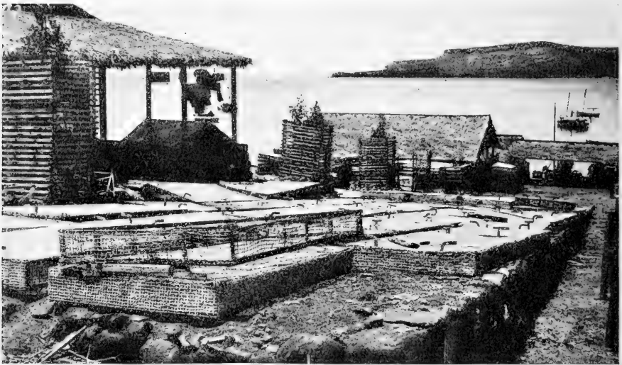
Fig. 37. Forms of wire apparatus for the protection and handling of pearl oysters laid out for growth.
