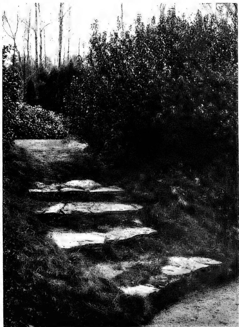
STEPS IN A ROUGH GRASS BANK; STONES CEMENTED AT FRONT.
