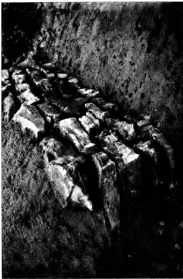
DRY ROCK-WALLING, SHOWING HOW THE STONES TIP BACK.
