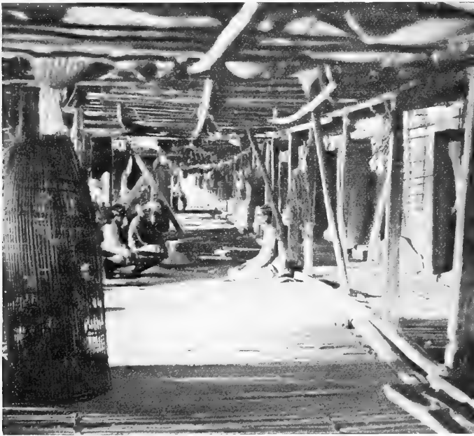
Fig. 33.—INTERIOR OF SEA-DYAK'S HOUSE.
