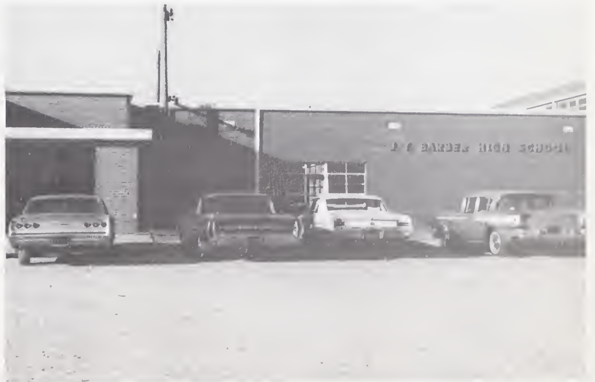
The Parking Area Was Completed.
