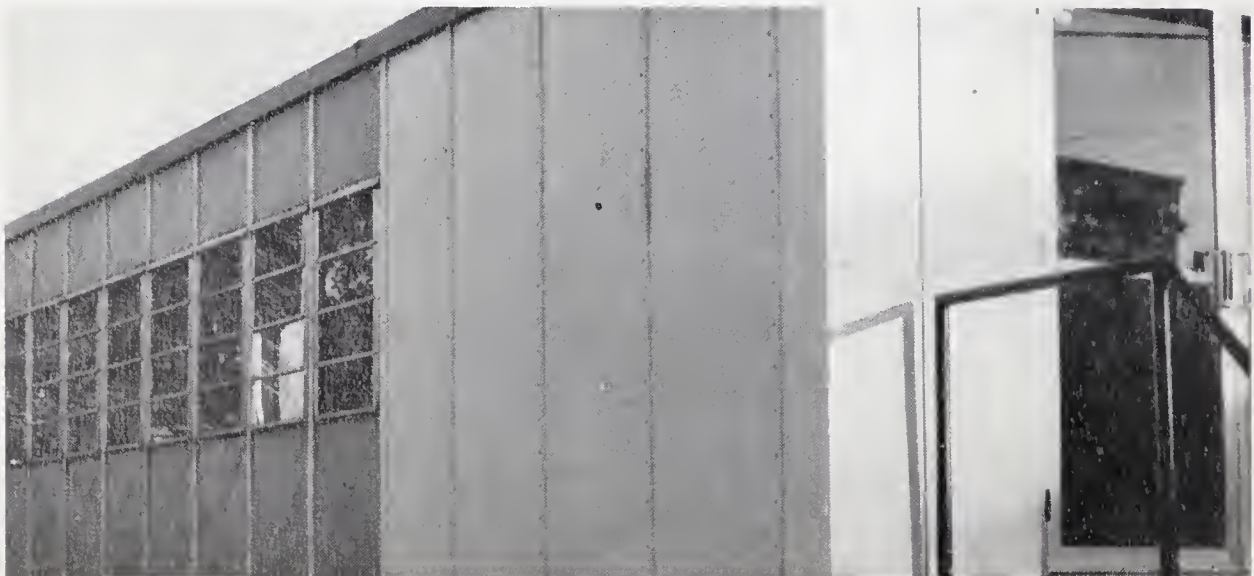
Mobile units were added to relieve the over-crowded conditions.
