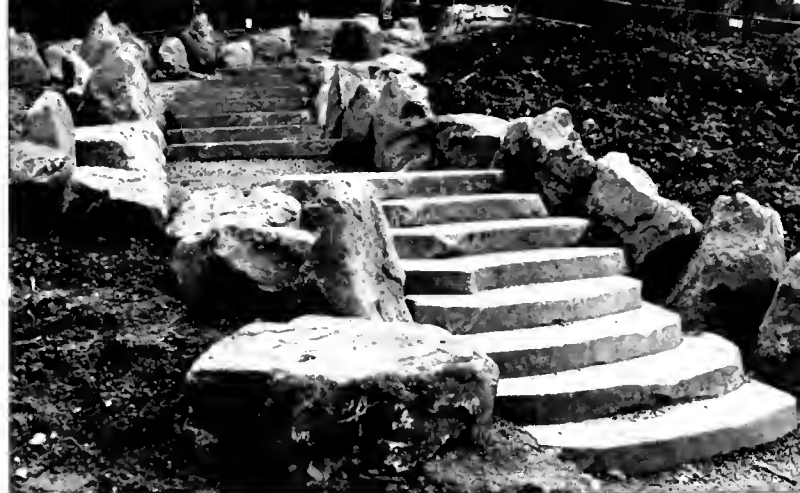
LEFT: This set of five steps are cut from a single boulder.
