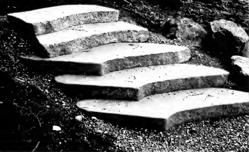
LEFT: This set of five steps are cut from a single boulder.
