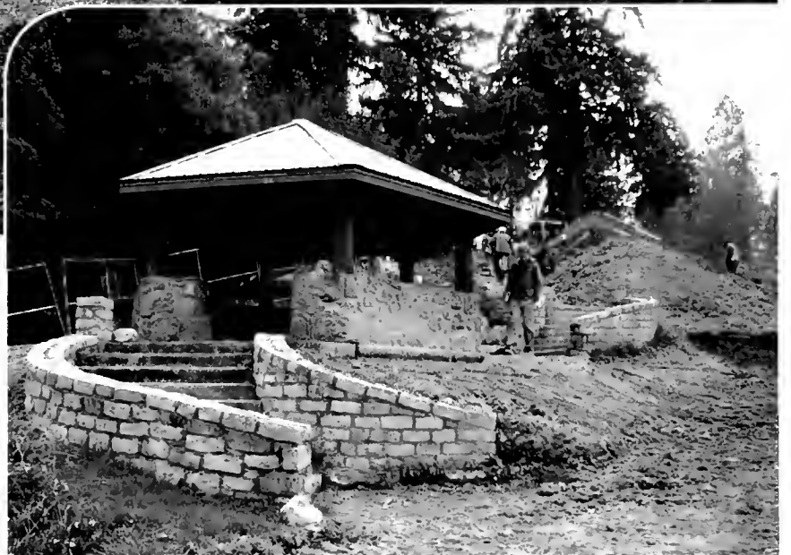
ABOVE: A new path down the slope creates access for pedestrians, wheel chairs and maintenance vehicles. The rock placed informally on the high side of the slope adds structure to the forest and a frame for the plants.
