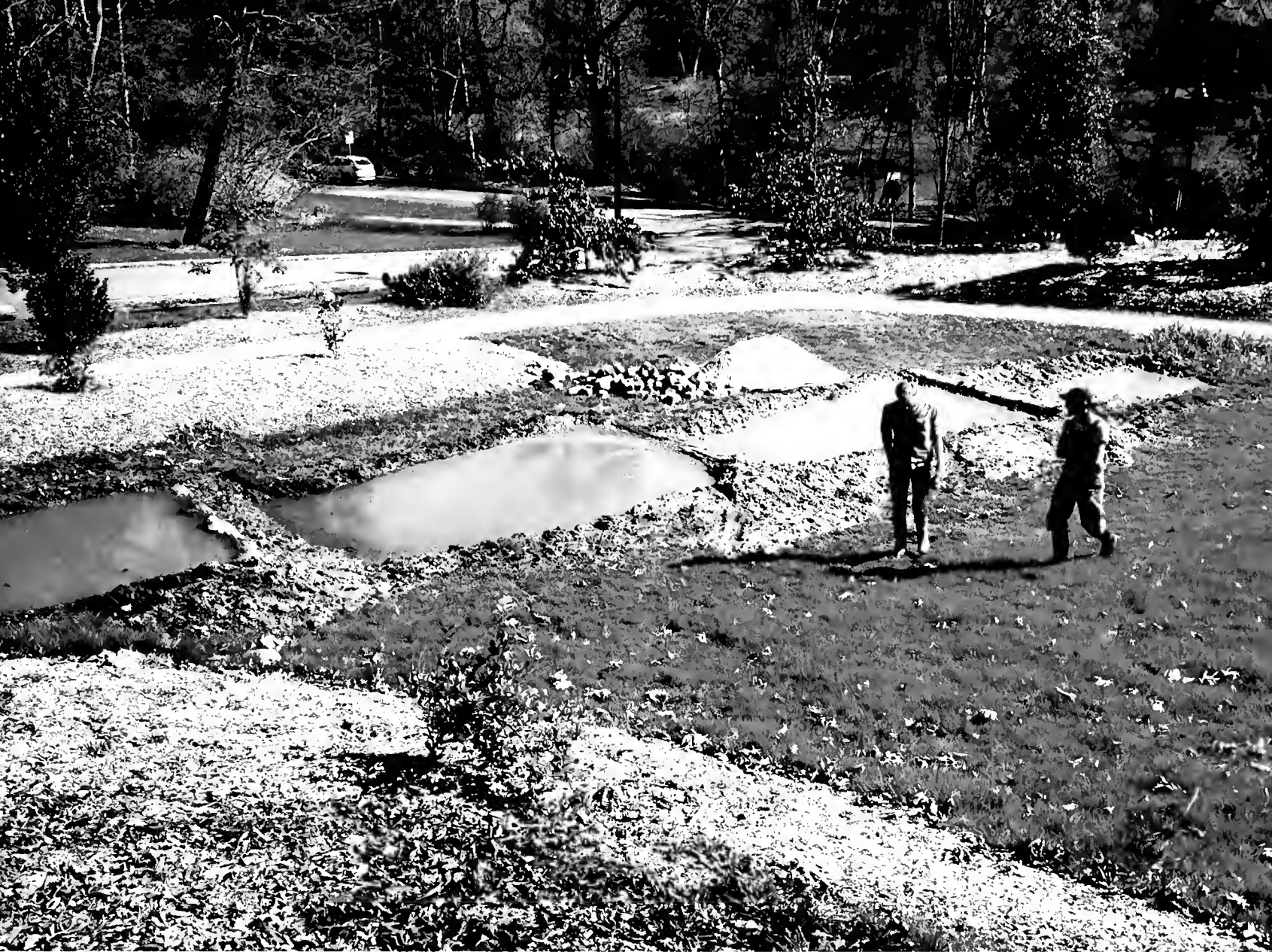
The step pool system ready for planting. (Photo courtesy Justin Bettis)
