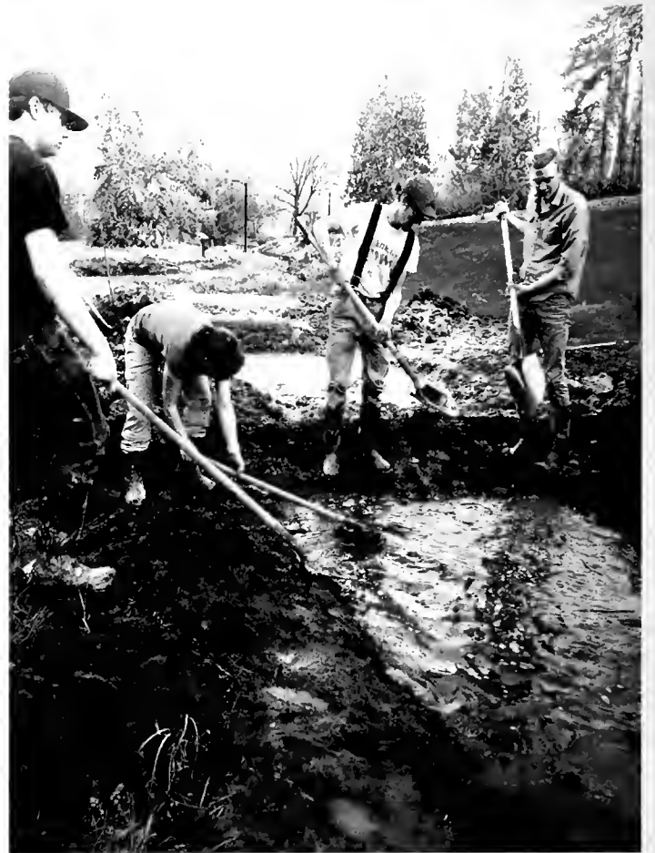
ABOVE: The students excavating soil from one of the weir system's step pools in spring 2013. (Photo courtesy Justin Bettis)
