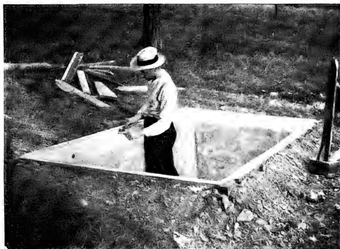
The tank is 8 x 4 ft. and was made of concrete. It cost $11.28 all told (For details see page 29)
