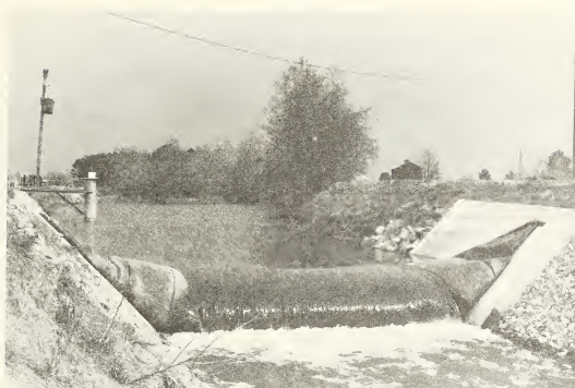
Fig. 5. Fabridam structure used for water control in a channelized stream.
