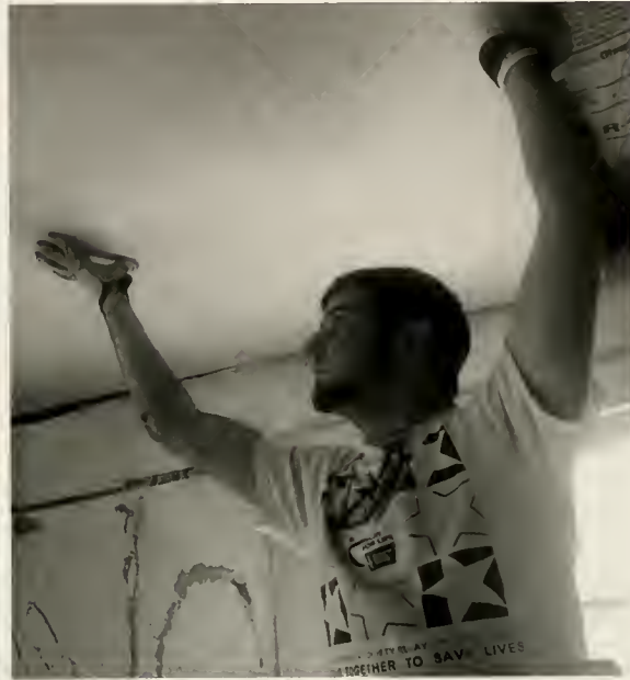
Below: Michael Scruggs hangs drywall in New Orleans.
