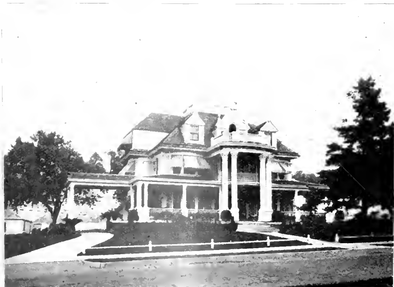
Residence of J. F. Wilcox, Council Bluffs, Iowa.
