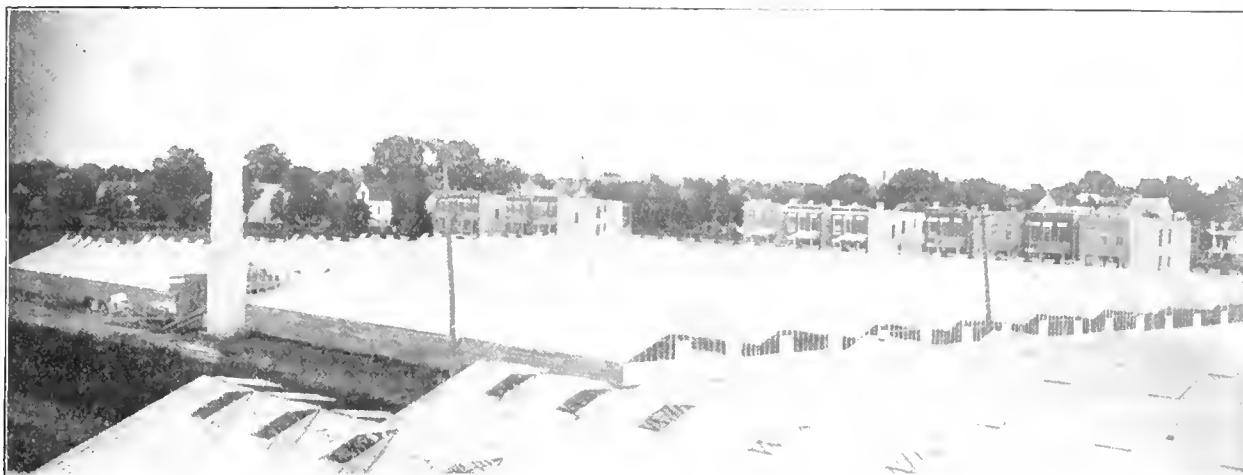
This is Mr. Reinberg's 1903 addition: Nine houses 27\frac{1}{2} \times 304 , 8\frac{1}{2} feet to the Garland Iron Gutter.
