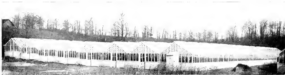
New Short-Span Greenhouses of A. Farenwald, the Liberty Grower, Hillside, Pa
