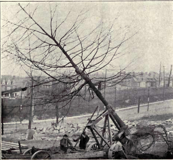
Moving large trees from the site of the new Carnegie Institute in Pittsburg to the lawn of Mr. W. L. Mellon, in the same city.
