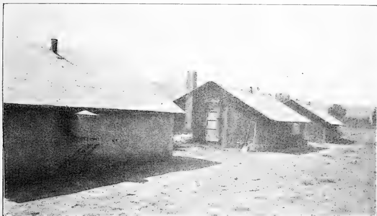
BROODER HOUSES, 14x20, DAVISON RANCH, ARLINGTON. EACH HOUSE BUILT TO CONTAIN 1500 CHICKS. WITH AUTOMATIC HEATER.
