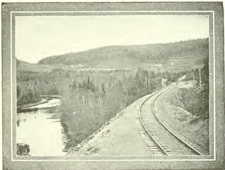
Between Fort Kent and Norcross.
