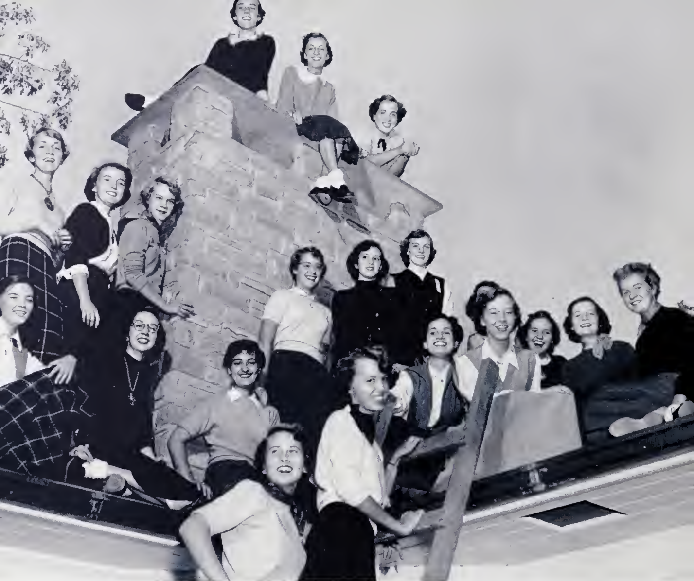
While the girls are usually content to just raise the roof, they seem to be having an equally good time lowering one. On the ladder are Anna Huffine and Doris Irvin. Seated, left to right, are Betty Sink, Nancy Williams, Chris Velonis, Ann Falk, Bettie Jane Upenreh, Bobbie Holler (partially hidden), Dava Cashwell, Sandra Bentz, Sue McEntire. Standing, left to right: Julie Hollowell, Jo Len Jamerson, Lillian Holland, Sally Durham, Frau Hosley, Kitten Barringer. On the chimney are Mary Helen Shelburne, Kathy Gryder, and Martha Jester.
